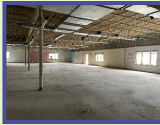
Before construction began—main entry way, former hallway, and future office space
